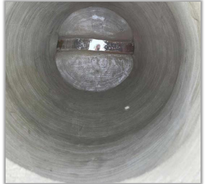
Manhole Rehabilitation & Relining
